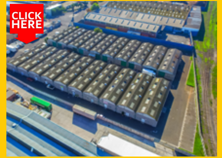
MALLEON INDUSTRIAL PARK 21 Christian Ave, Freehold
